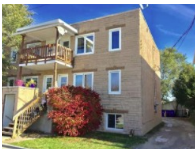
6 logements Construction : 1953 104 East, Gatineau (Town Side) Transaction : 2019-06-18, 523 500 $ (87 250 $/log.)
